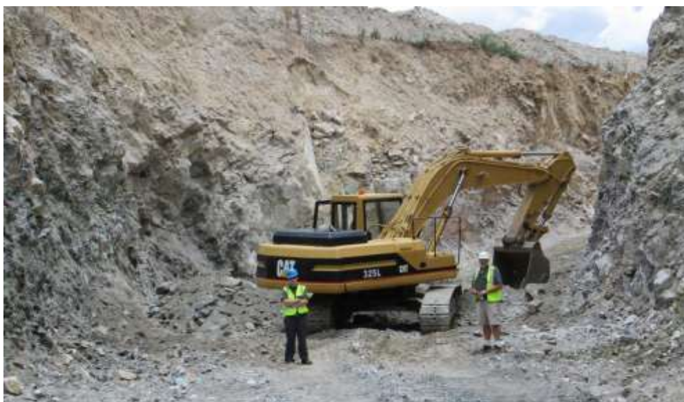
Figure 3. Excavating the oxide copper bulk sample pit, November 2012
